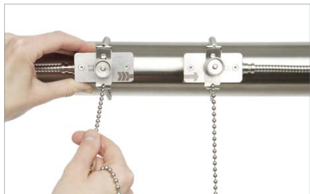
Transducers mounted using chains and clips
